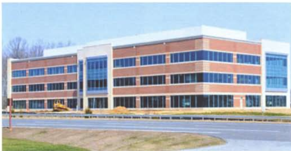
Office Building at North Gate Business Park
