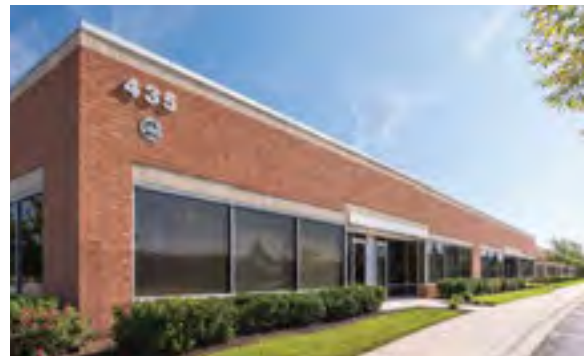
Single-story class 'A' office exterior
